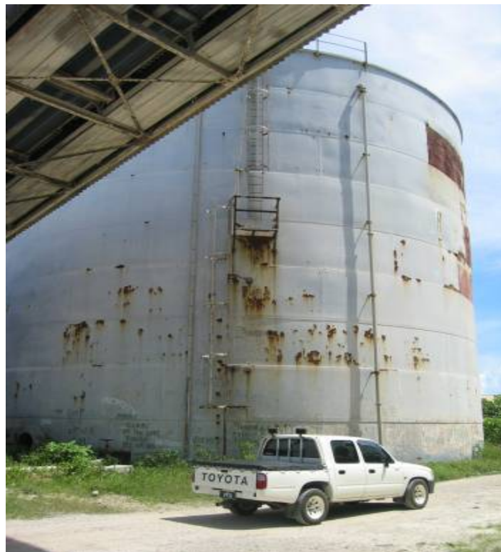
Decommissioned Water Storage Tank B12
