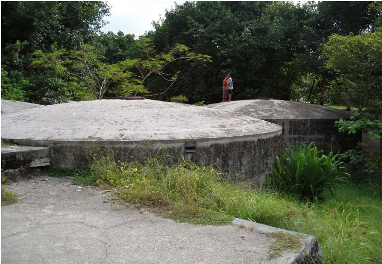
Nauru – Reinforced concrete water storage tanks (derelict)
