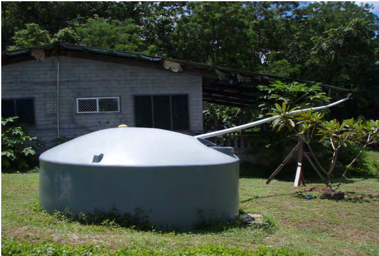
Plastic water storage tank emplaced partially below ground level, Buada, Nauru.
