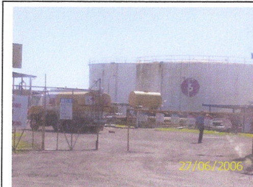
Figure 15: Petroleum storage facilities must adhere to national and international safety and quality standards.
