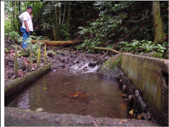
Unprotected Water Intake point
