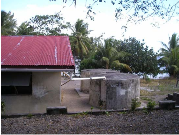
Figure 9 Community water tanks
