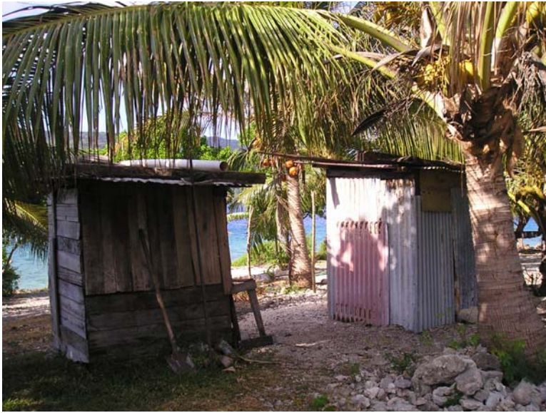
Figure 1 Buildings are typically close to the coast on Lelepa Island
