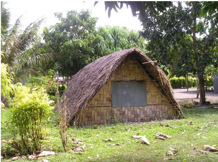
Figure 3 Local 'A frame' style house with wild cane roof
