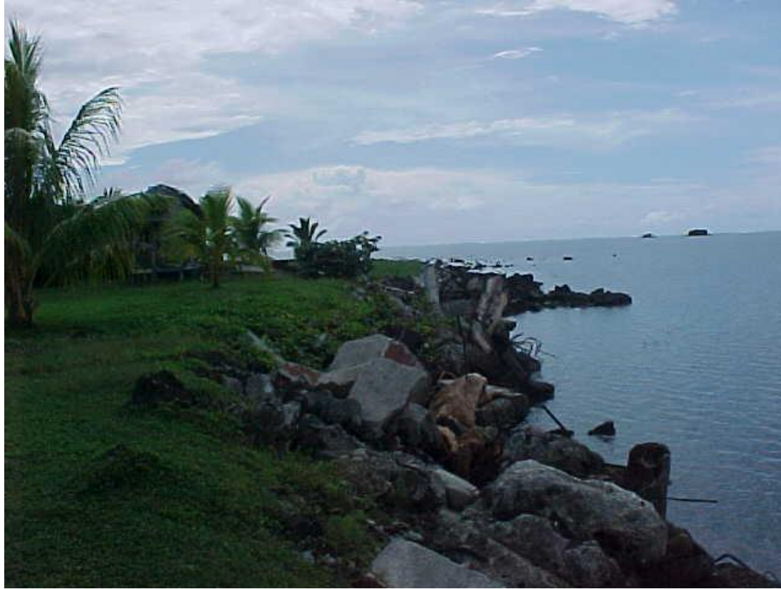
Seawall and reclamation at Savaiian Hotel and adjacent property.
