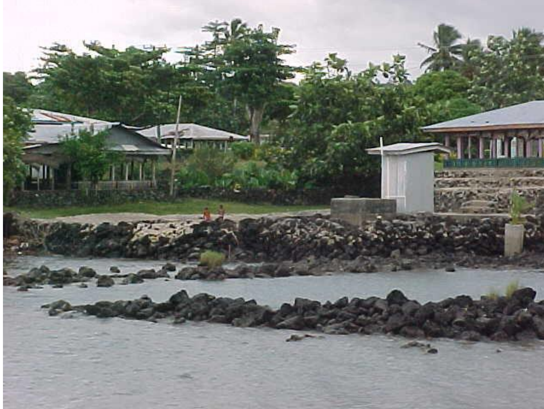
Lagoon inlet to Vaitele Pool. Women's Committee House behind to the right and toilet in foreground.
