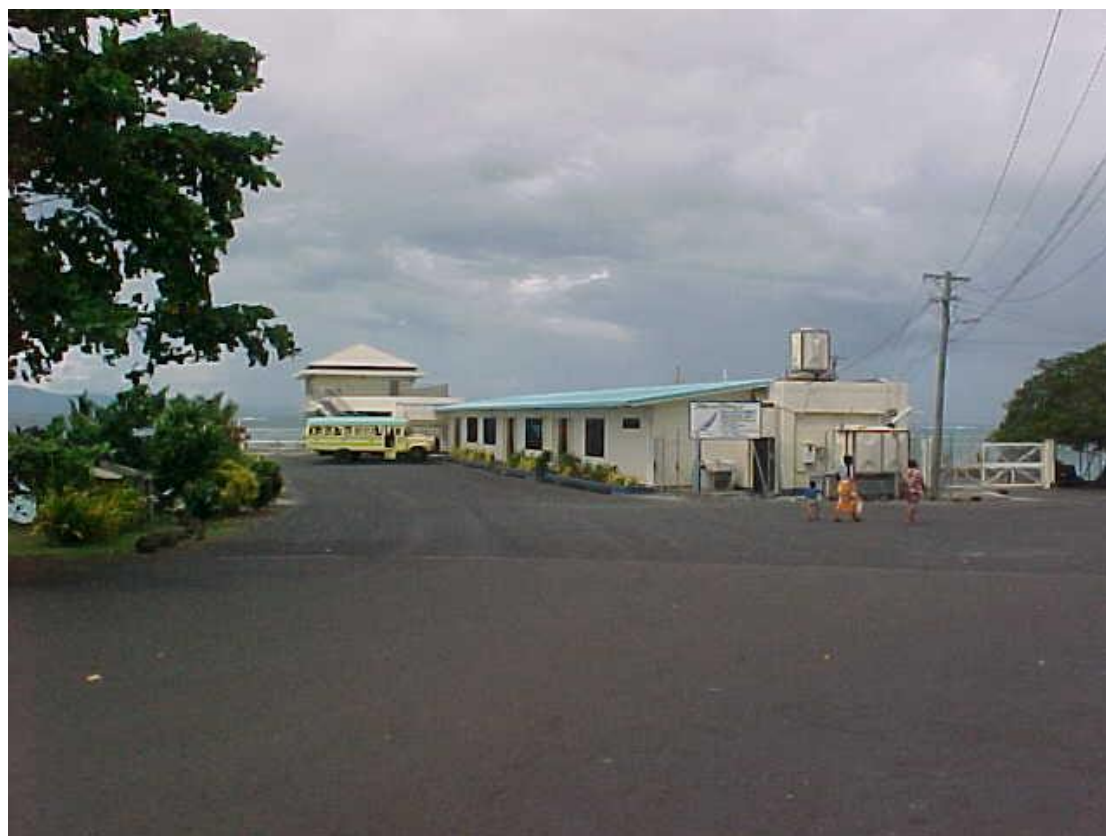
Salelologa wharf. Recently constructed substantial buildings made from concrete block.
