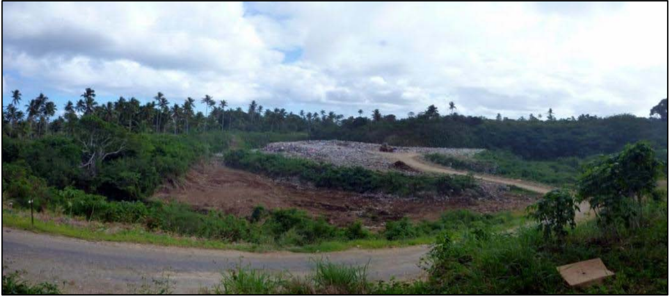
Photo 4: Tapuhia Landfill: view of cell 1 (with rubbish), and cell 2 (under preparation)
