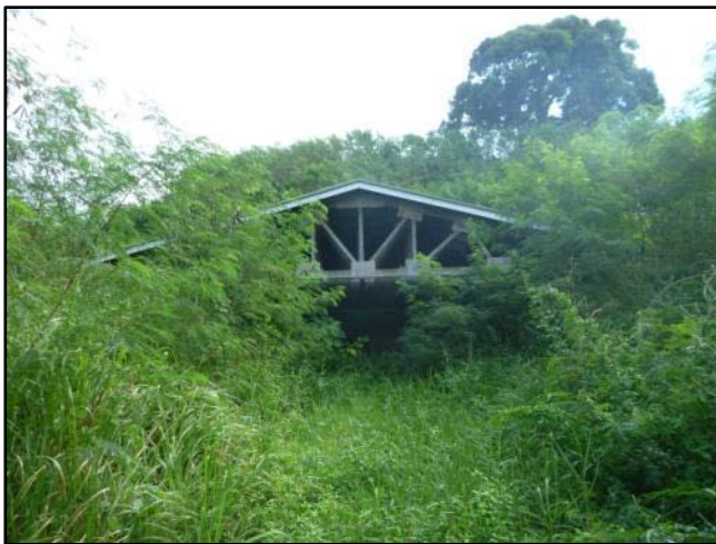
Photo 5: Disused hazardous waste storage/disposal area
