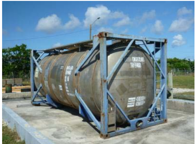
Photo 15: Tonga Power's 24,000 litre tanktainer in a bunded area
