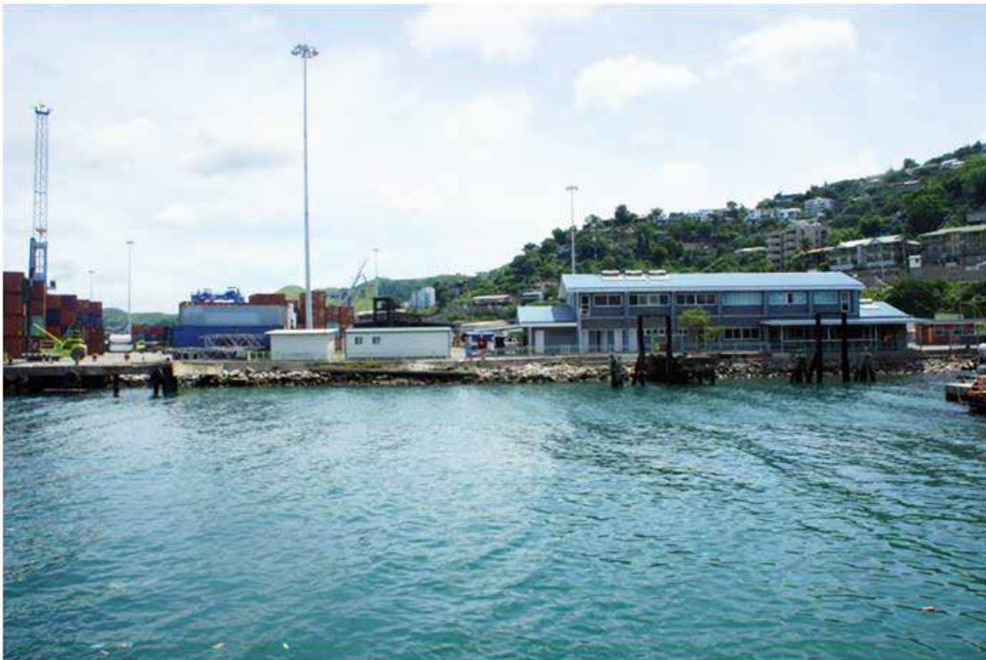
Figure 5: Eastern view of Laurabada Wharf, Container Terminal, PoM
