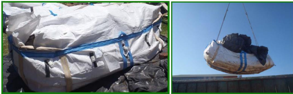
Photos 5 & 6: Asbags in use
