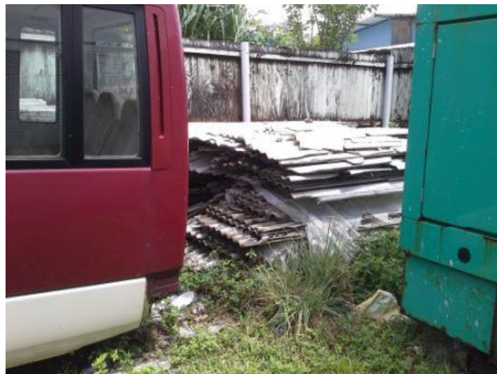
Photo 2: Asbestos sheets at the College of MI
