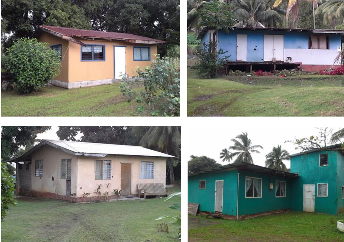
Photos 5-9 – Typical Residences with PACM Cladding
