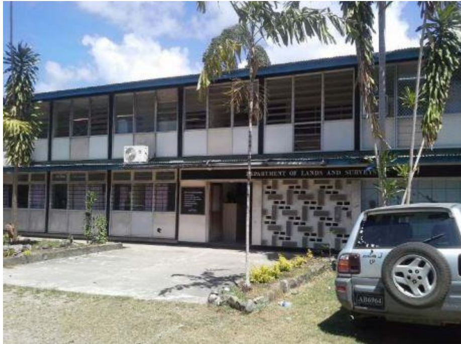
Photo 3: Lands & Survey Building – AC Panels
