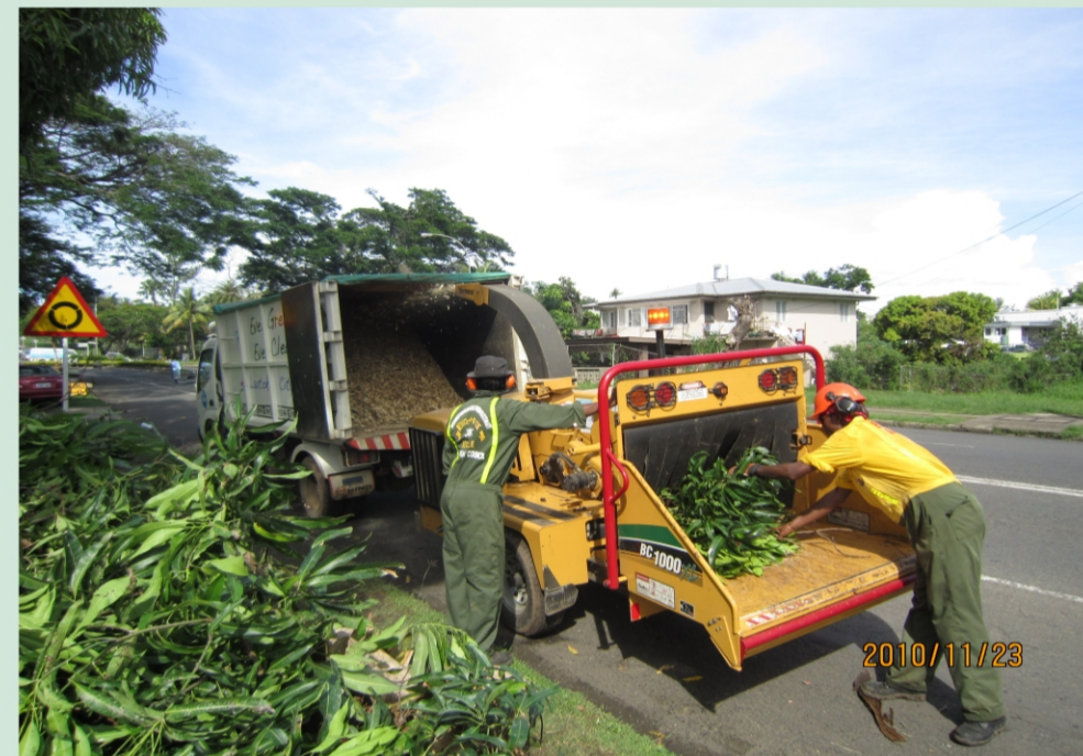
(Chipping at site)
