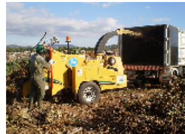
Shredding work at final disposal site (LCC)
