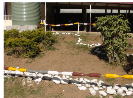
PET bottle chains for fencing in compound
