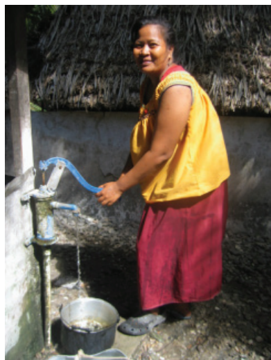
Protected well water collected and stored in pots at the point of use, Bikenibeu
