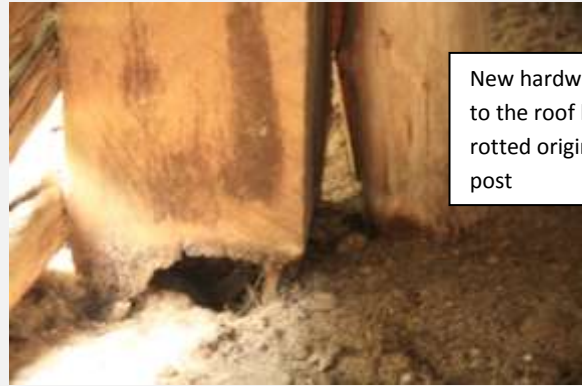
b. Posts in 'white man's' houses rotted away and needed to be supported using local hard wood shown here.
