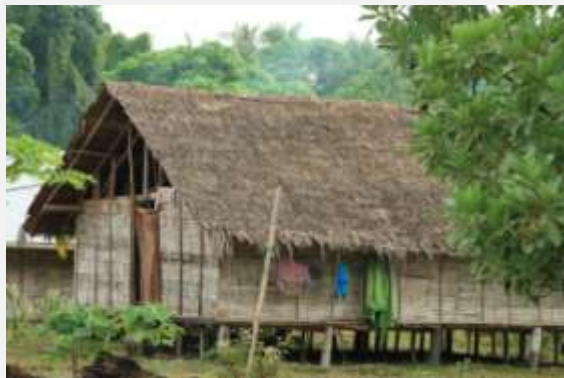
c. Some households chose to build their houses on stilts at the new site, Lirak
