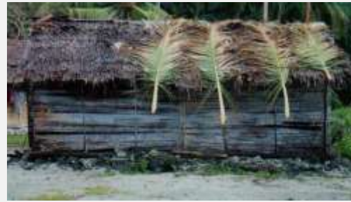
b. House perched on rocks to accommodate small levels of flooding (Phillip nd)
