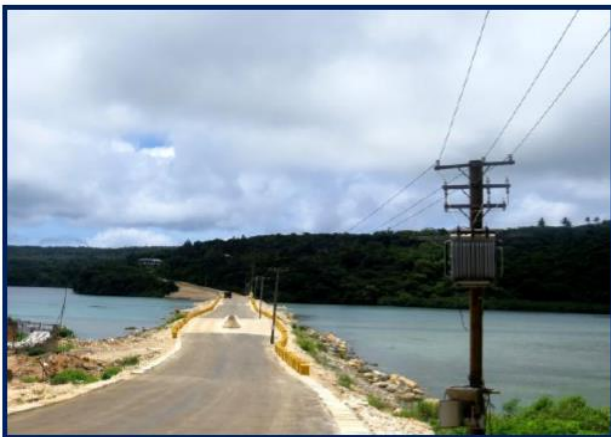
Photo 11: TPL Distribution Grid connecting two Islands in Vava'u
