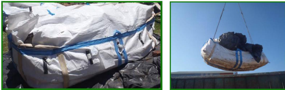
Photos 8 & 9: Asbags in use
