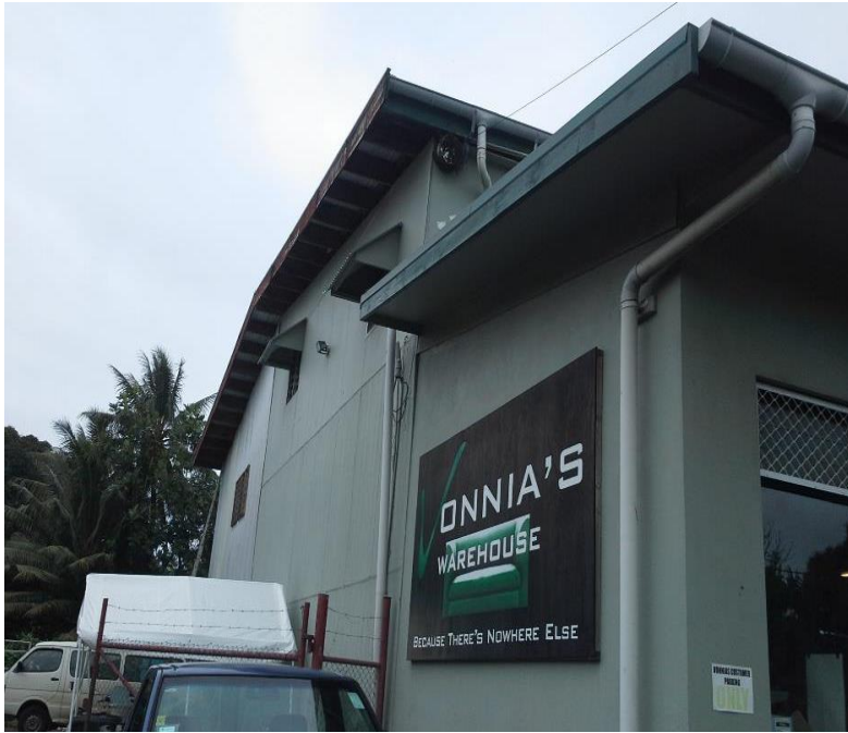
Photo 6 - Typical Commercial Building
