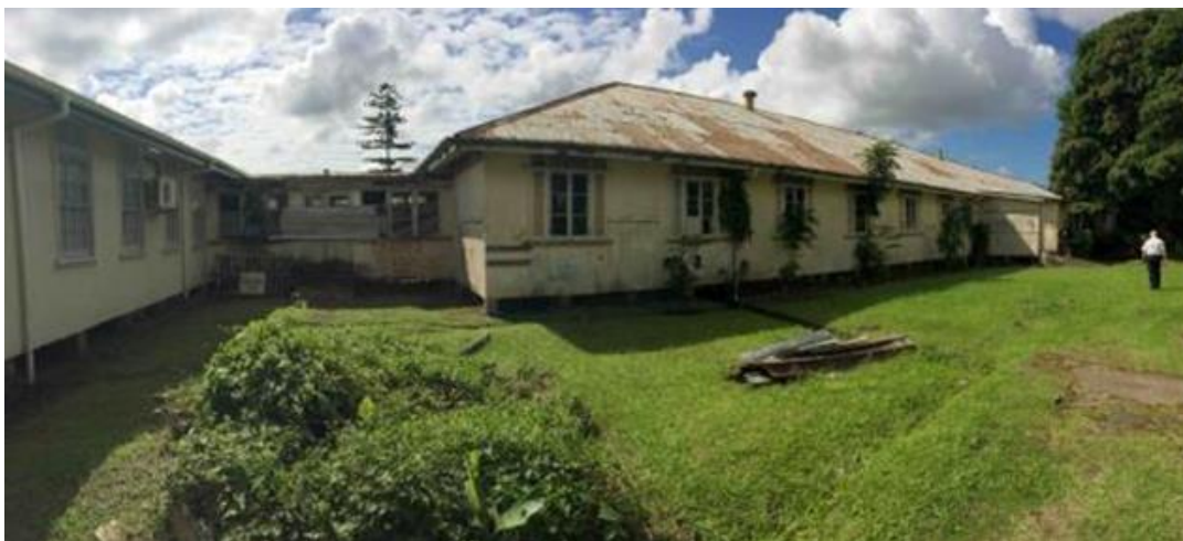
Photo 9 – Old Ward 5 Building, Tamavua-Twomey Hospital
