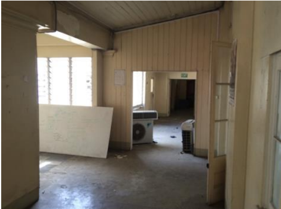
Photograph 3: View of 1 st floor 16 July 2014.
