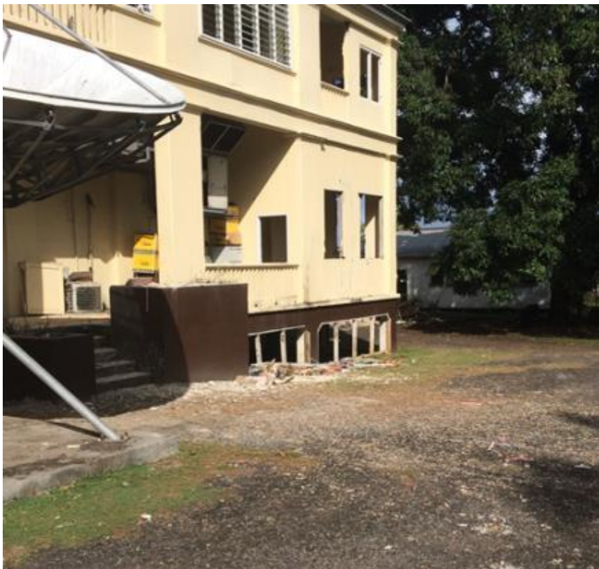
Photograph 6; acm vinyl floor tiles on ground adjacent to north facing façade
