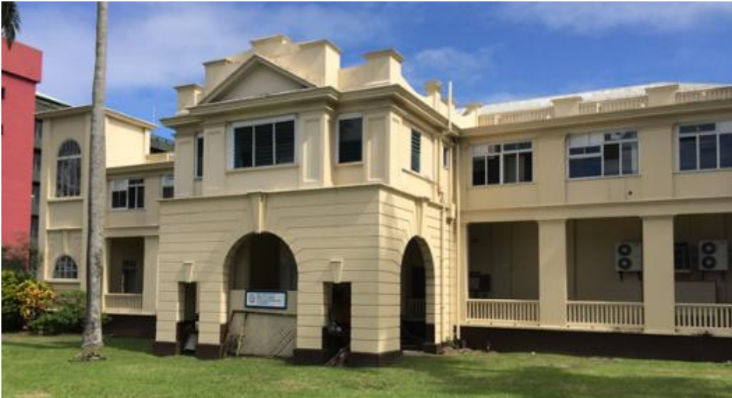
Photograph 1: View South West of St Stephens Building 16 July 2014.
