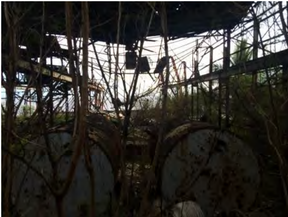
Photograph 21: Warehouse 7 by wharf – another badly damaged building with ACM scattered across site.
