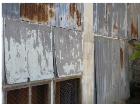
Photo 2 – Rear of Old Powerhouse
