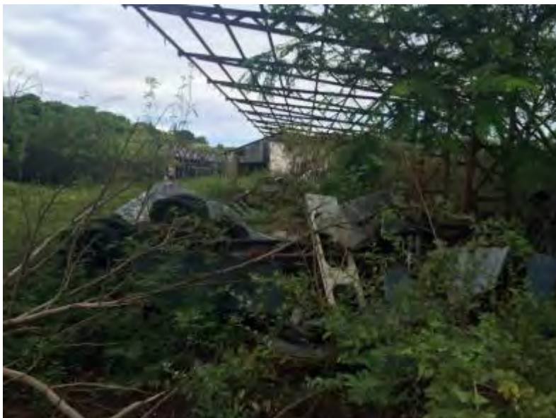
Photo 17: Former mechanical repair workshop building with no cladding or roof
