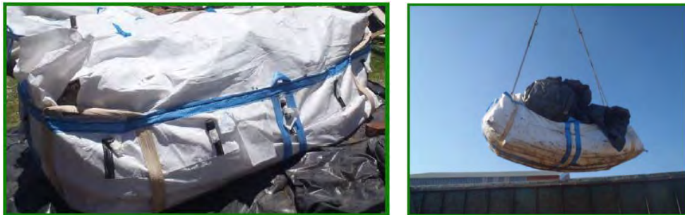
Photos 27 & 28: Asbags in use
