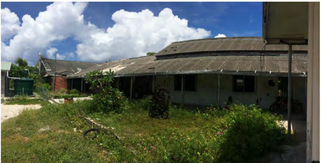
Photograph 2: Banaba Hospital – acm roof.
