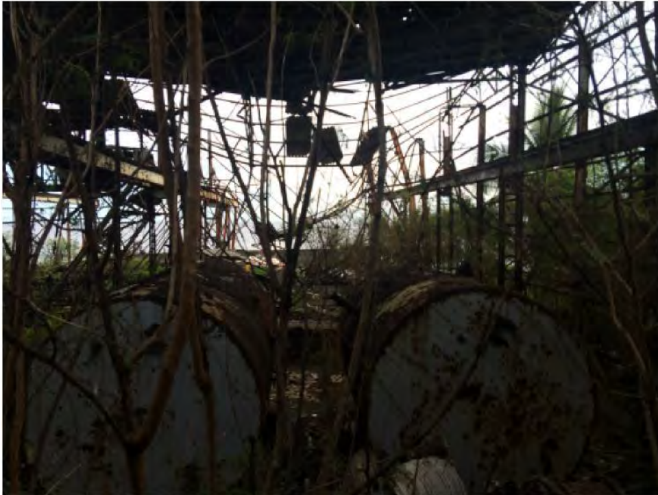
Photograph 15: Warehouse 7 by wharf – another badly damaged building with acm scattered across site.
