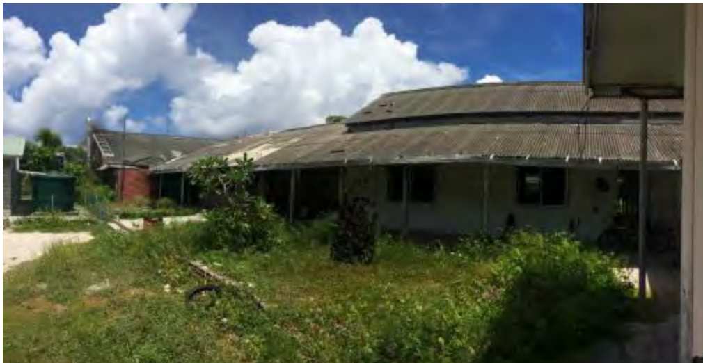
Photo 8: Banaba Hospital – ACM Roof
