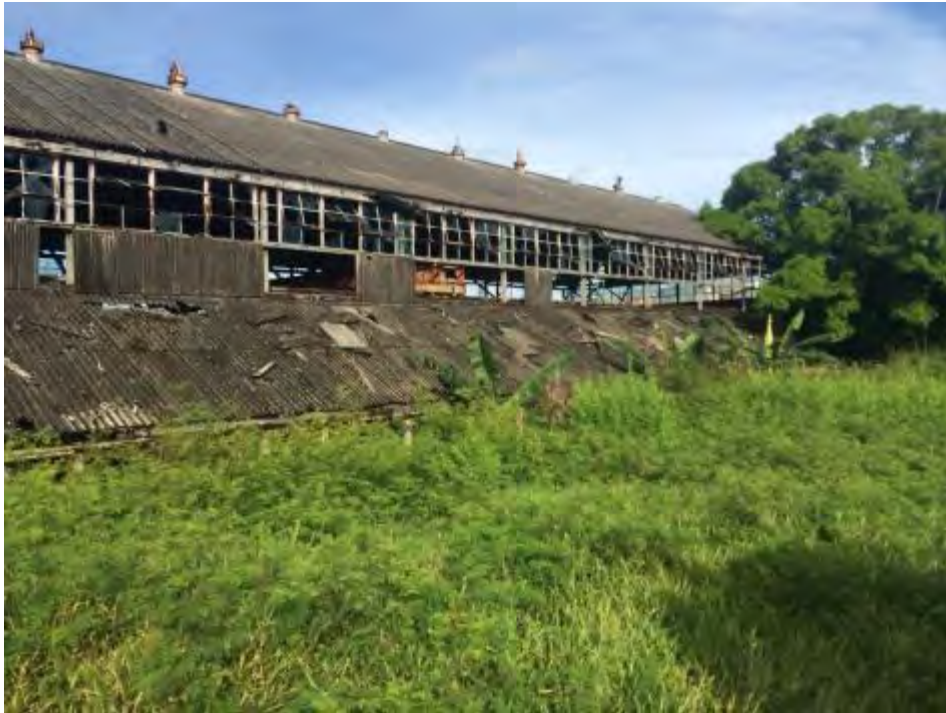
Photo 11: Banaba former power house. ACM Roof
