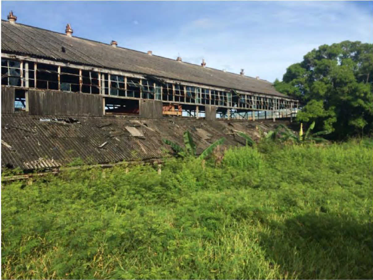
Photograph 5: Banaba former power house. pacm roof.
