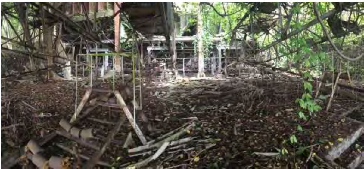
Photo 16: Former phosphate processing plant. View towards hoppers at rear
