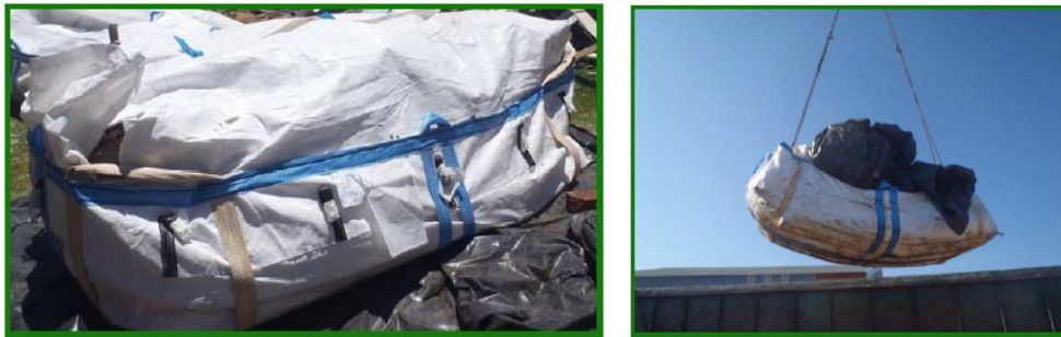
Photos 10 and 11: Asbags in use
