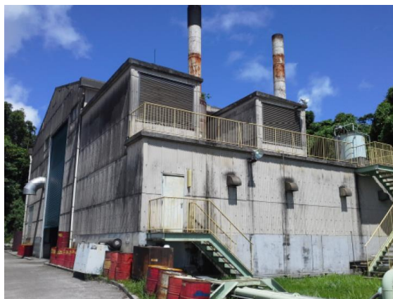
Photo 1 – Malakal Power Station New Generator Building
