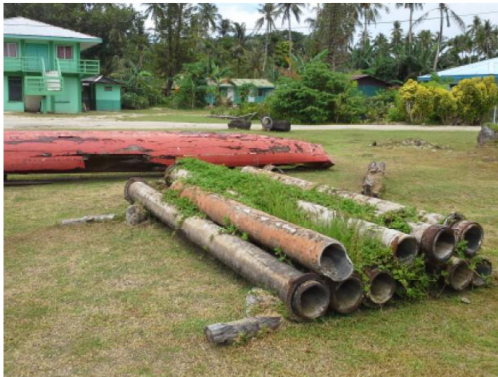
Photo 4 – Old Pipes in reserve in Ngiwai Village
