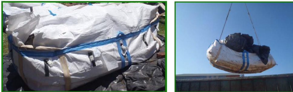
Photos 17 and 18: Asbags in use
