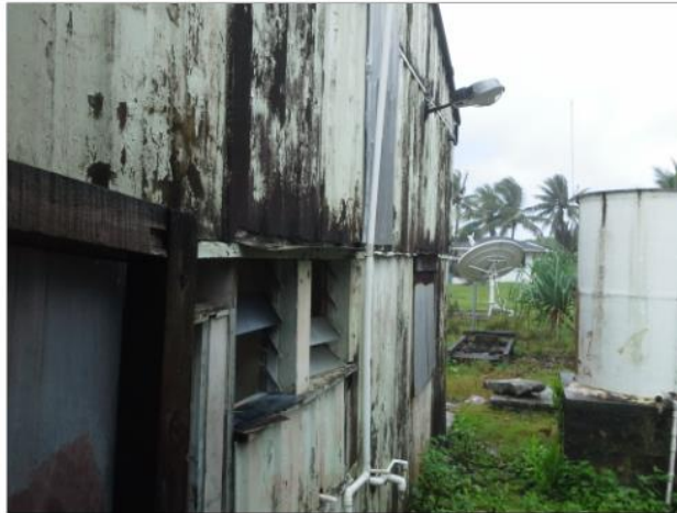
Photo 2: Wall cladding on the former power station
