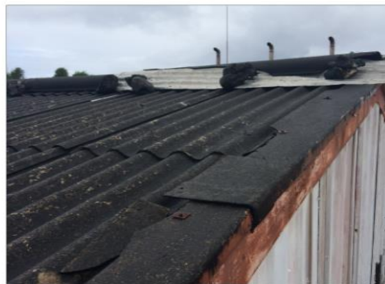
Photo 3: Asbestos roofing material on the former power station
