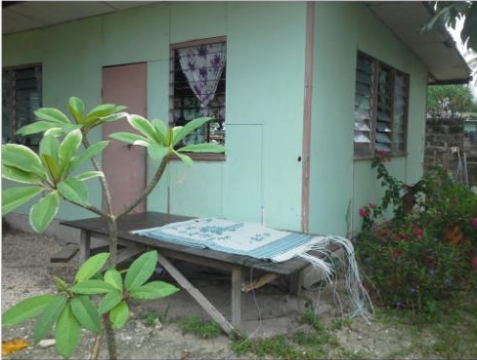
Photo 1: typical structure in Funafuti showing fibre board cladding
