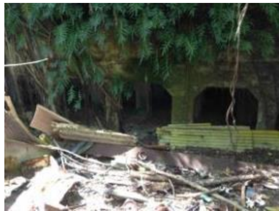
Photo 16 – Tunnel Reported to Contain More Bags
