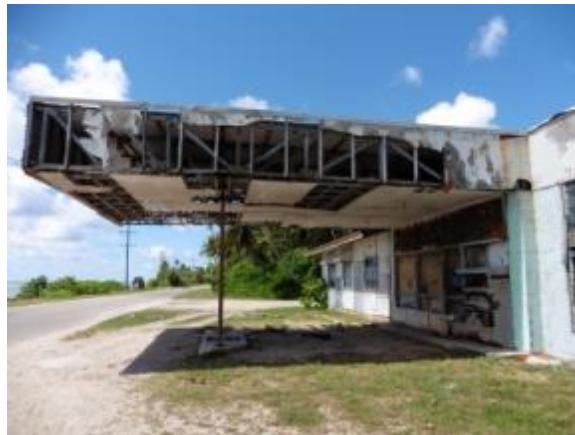
Photo 70 - Abandoned Petrol Station
