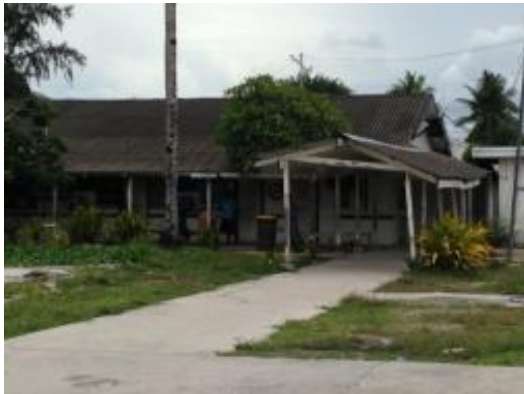
Photo 15 – Old Hospital Block
