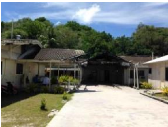
Photo 10 – Burnt Part of Hospital
