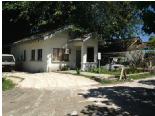
Photos 5-10 – Six Typical Houses with Asbestos Roofs and Possibly Asbestos Cladding
