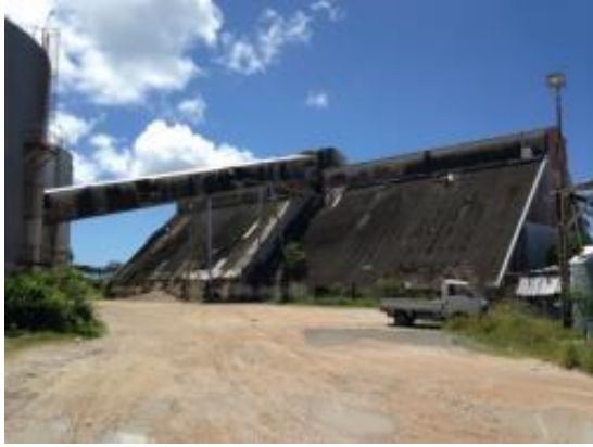
Photo 42 - Phosphate Storage Bin by Sea
