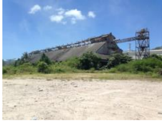
Photo 43 - Old Phosphate Storage Bin by Sports Field
