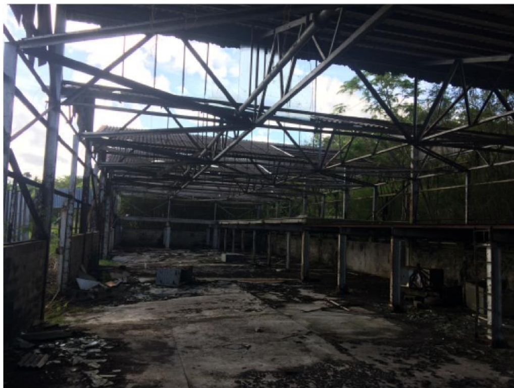
Photograph 16: Warehouse 3 – badly damaged pacm roof and walls.
