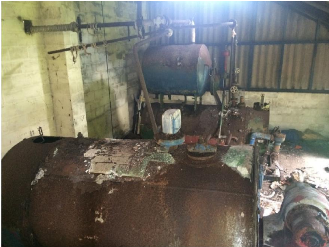
Photograph 7: Residential property 18, boilers with pacm lagging.
