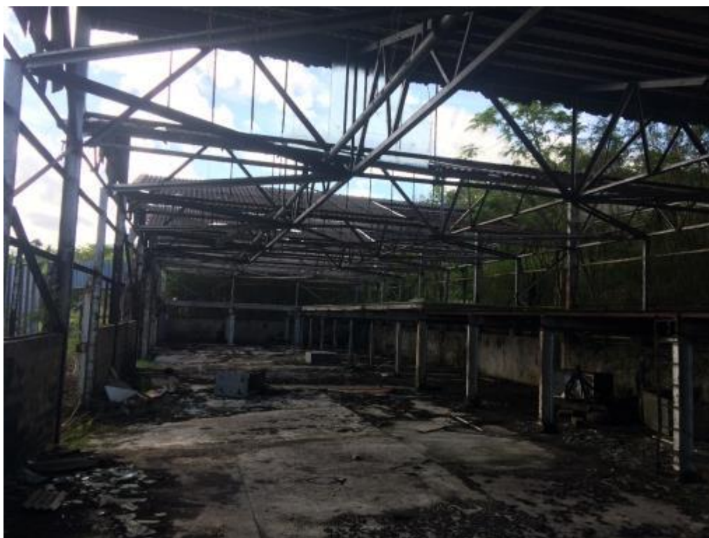
Photo 22: Warehouse 3 – badly damaged ACM roof and walls.
