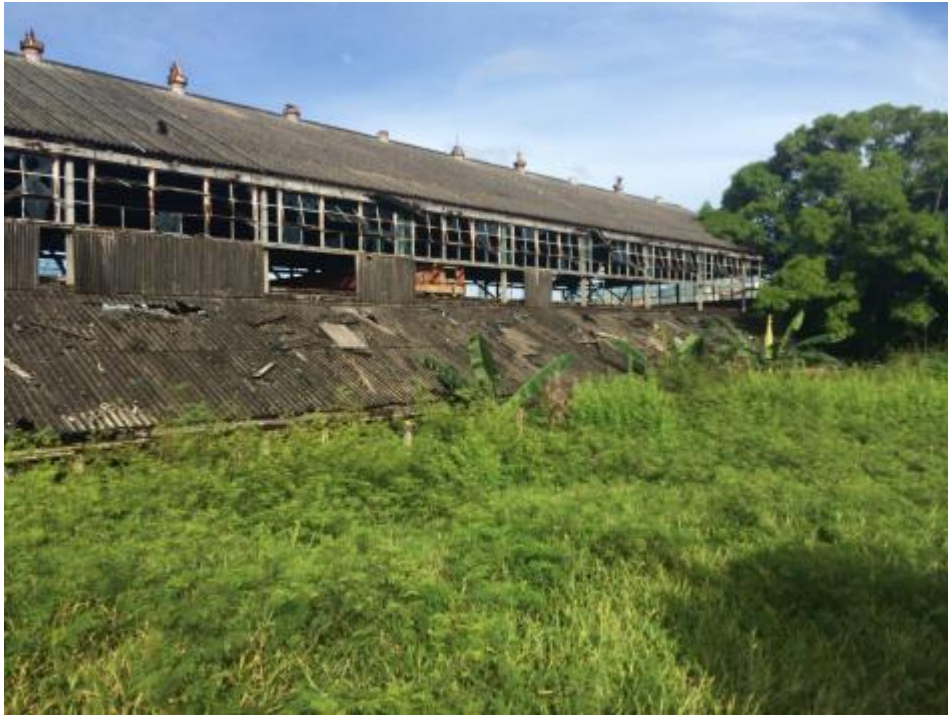
Photo 11: Banaba former power house. ACM Roof
