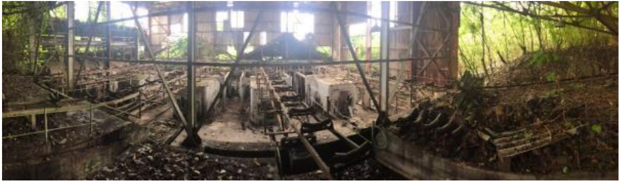
Photo 15: Former phosphate processing plant. In dis-repair with significant ACM scattered across entire site.
