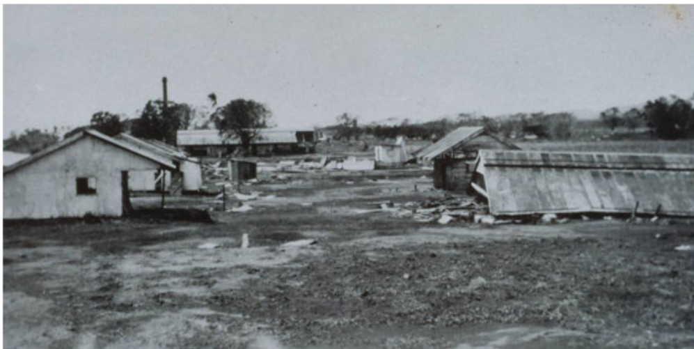
Destroyed buildings at Rarawai Mill, Ba, after the disastrous flood of February 1931. The loss of life from this event exceeded 200 people, mostly in the Ba and Lautoka districts. (Photo source: CSR, 1931).
