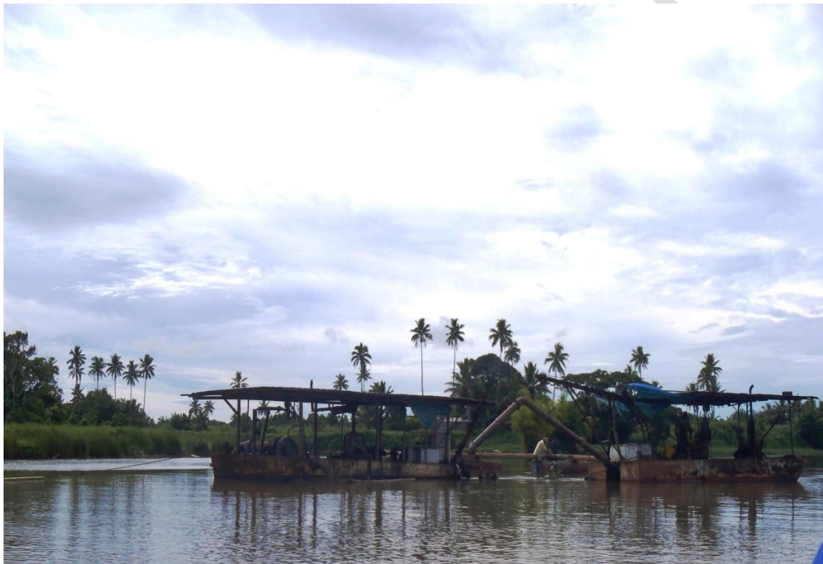
Dredging at the Rewa River.
