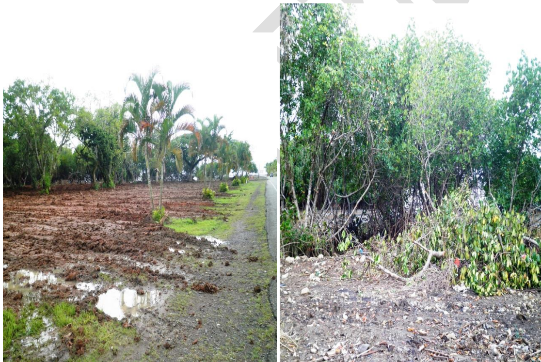
Mangrove are cleared to make recreational park in Suva.
