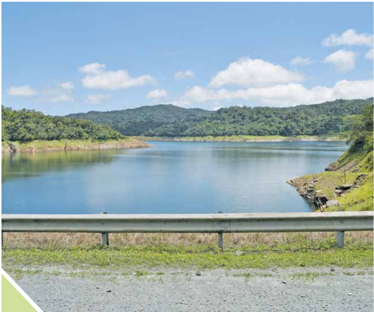
Monasavu Hydropower reservoir
