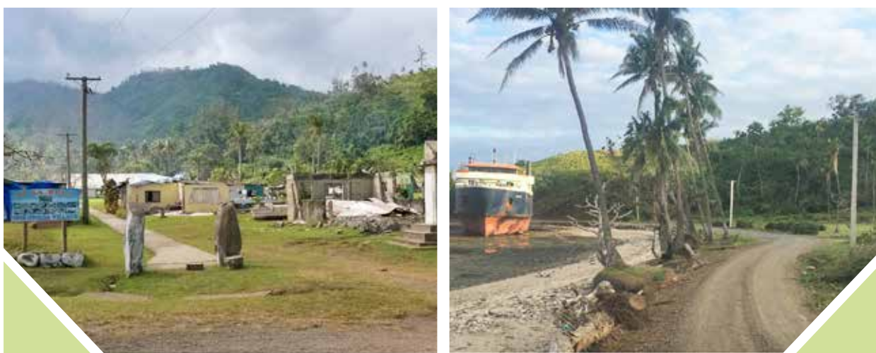
Damage from TC Winston on Ovalau Island in 2016
