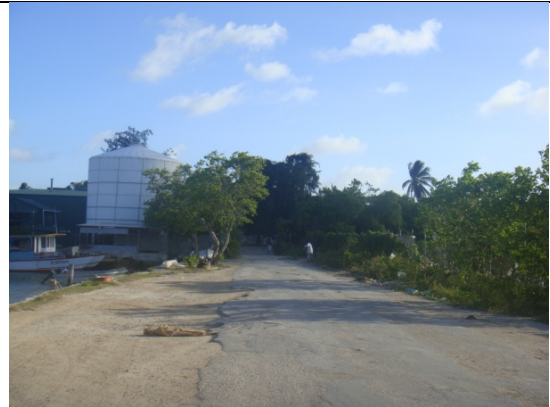
Looking back along secondary access road
