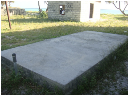
Cistern, eastern side of old desalination building
