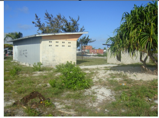
Old desalination plant building from ocean foreshore
