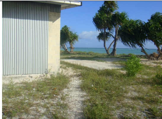
Slab over cistern at rear of the old desalination plant building
