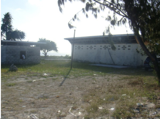
Site looking from east
