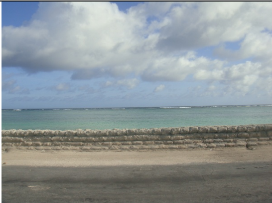
Looking across sea wall at ocean side
