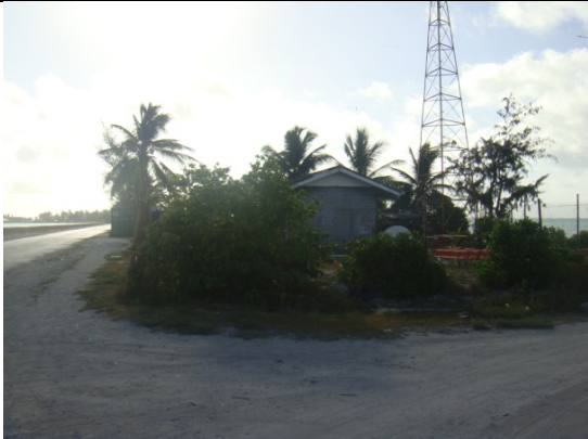
TSKL storage site and fence
