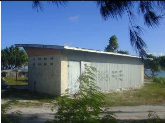
Old desalination plant building
