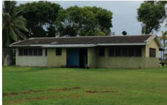
Honey Processing Building Roof
