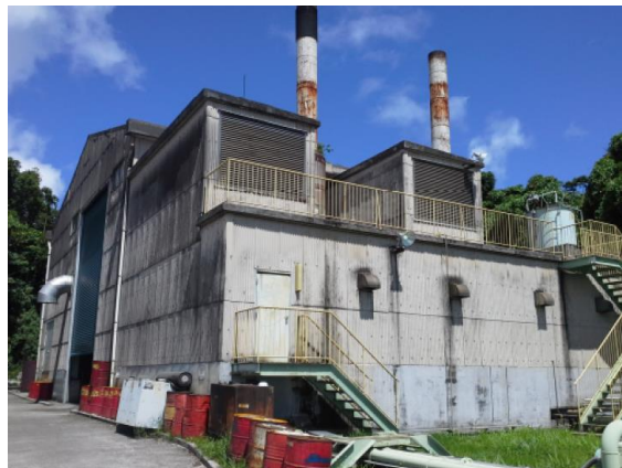
Malakal Power Station New Generator Building
