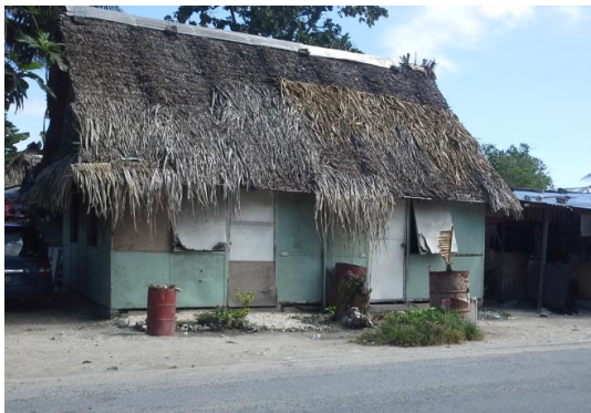
Kiribati Houses with Asbestos Cladding
