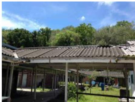
Hospital Parapet Roof
