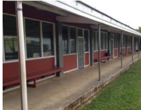
Secondary School Cladding
