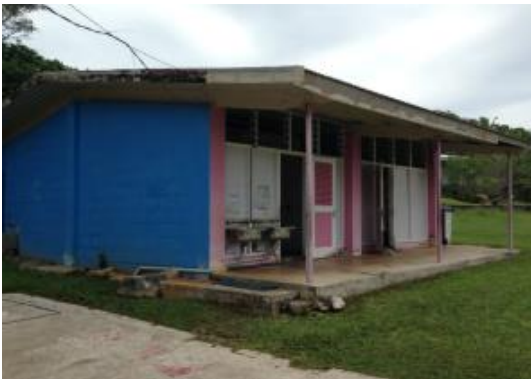
Primary School – Cladding and Soffits
