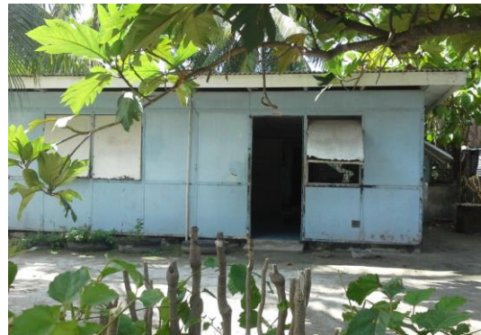
Kiribati Houses with Asbestos Cladding
