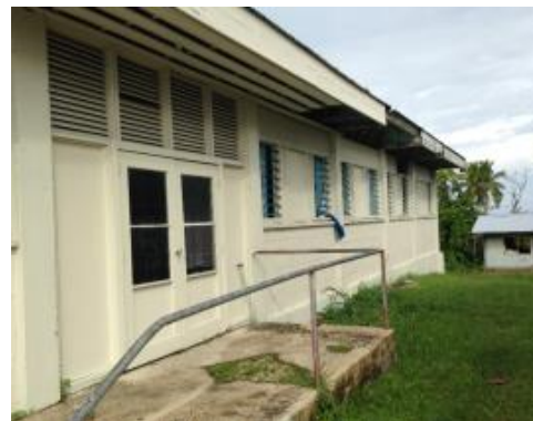
Alofi South Hall Cladding
