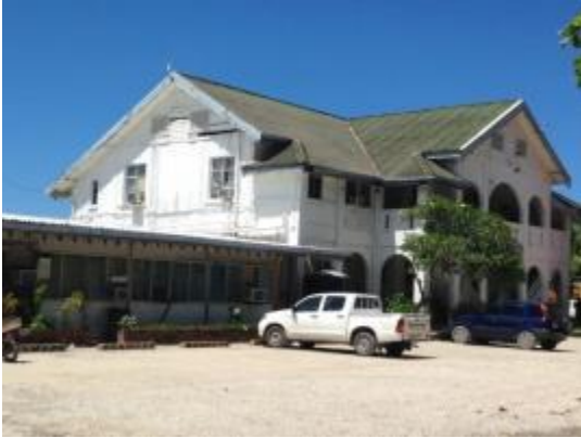
Central Office Building
