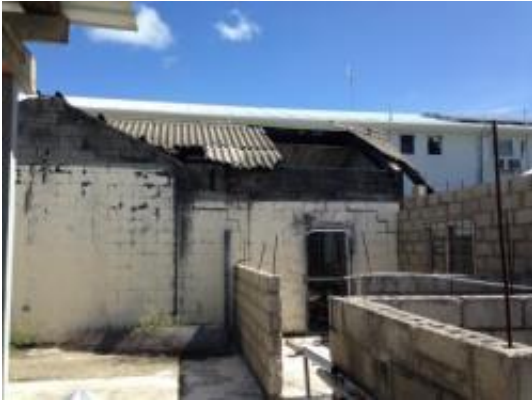
Prison Asbestos in Burnt Area including Asbestos Debris
