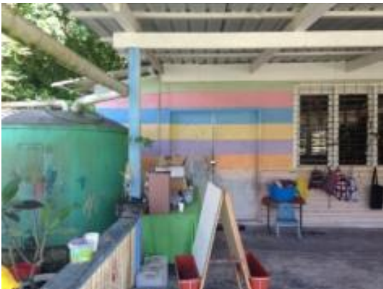
Nibok Infant School Asbestos Cladding and Suspected Ceiling
