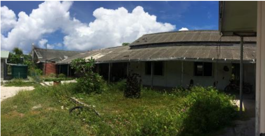
Banaba Hospital – ACM Roof
