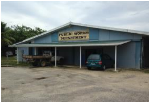
Public Works Department Cladding
