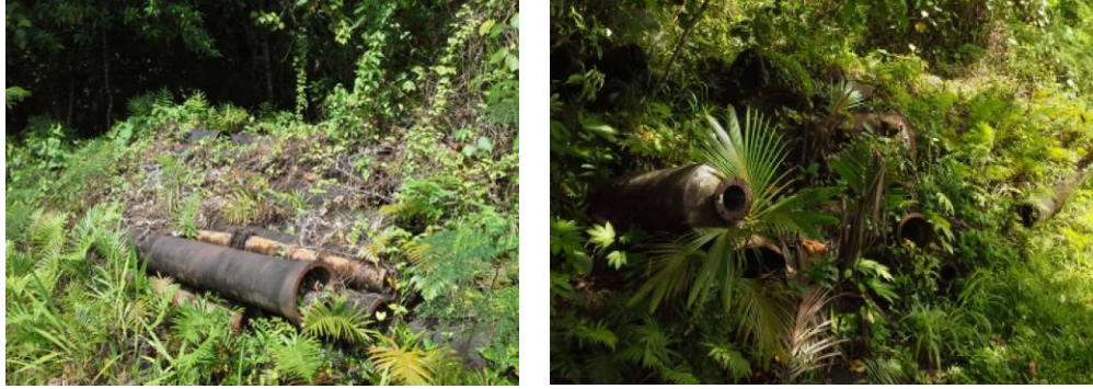
Old Asbestos Pipes at Palau Water Treatment Plant
