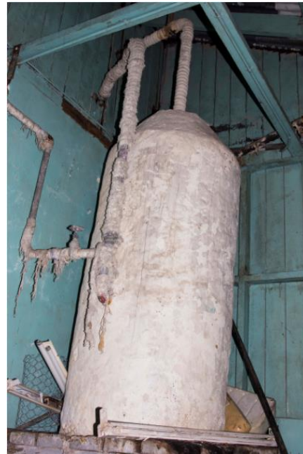
Tamavua-Twomey Hospital Lagging on Pipes and Hospital Boiler
