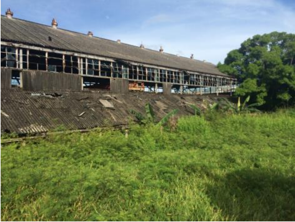
Banaba former power house
