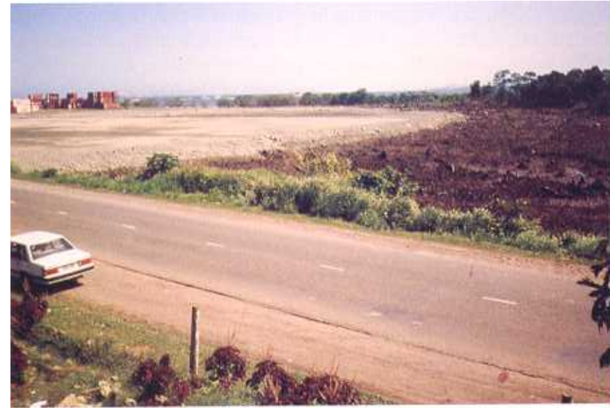
Plate 13. Reclamation of mangroves for use as a container storage area near the Port of Suva, Walu Bay, Fiji. Note a narrow fringe of mangroves left along the exposed side of the reclaimed area to protect the fill from wave action.
