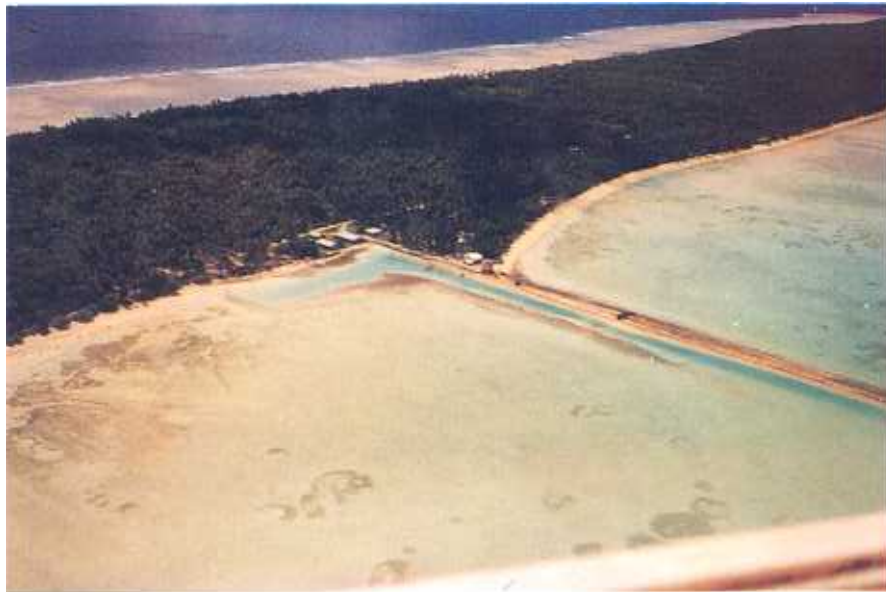
Plate 22. A coral rubble mole in Abemama, Kiribati, has acted as a groyne, accumulating sand on the updrift side (right) and causing shoreline erosion along several hundred metres of beach on the downdrift side (left).
