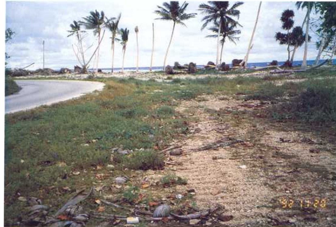
Plates 25 and 26. The present solid waste disposal site (rubbish dump) being retained by a wall constructed of gabion baskets on the ocean side reef flat of Majuro Atoll, Marshall Islands. Note the narrow reef flat and the position of the gabions virtually at the reef edge at the top right of Plate 25, above. The end result is useable reclaimed land (Plate 26).
