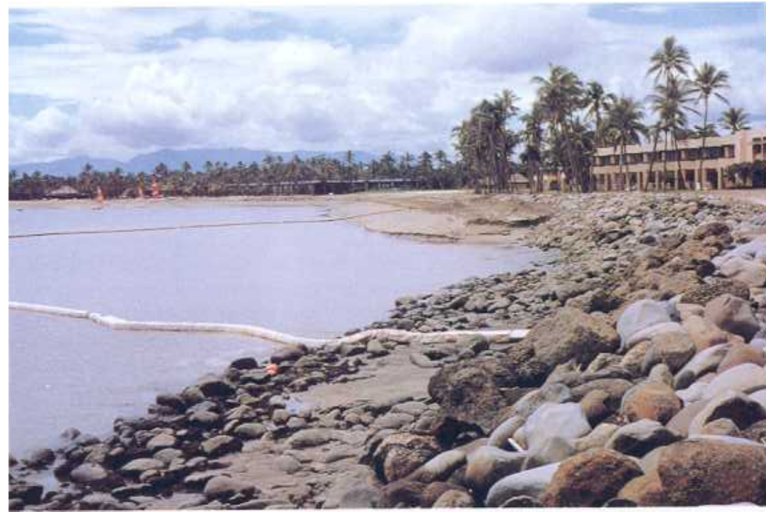
Plate 34. Artificial replenishment of beach in front of the Regent of Fiji is being carried out by trucking sand to replace that lost by erosion. The erosion problem was caused by a groyne which blocked off the natural supply of sand to the beach.
