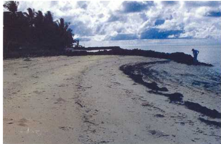
Plate 41. The groyne has been built out across the beach to trap sand prior to making a reclamation. Sand will be lost to the beach on the other side of the groyne, and beach erosion will take place.
