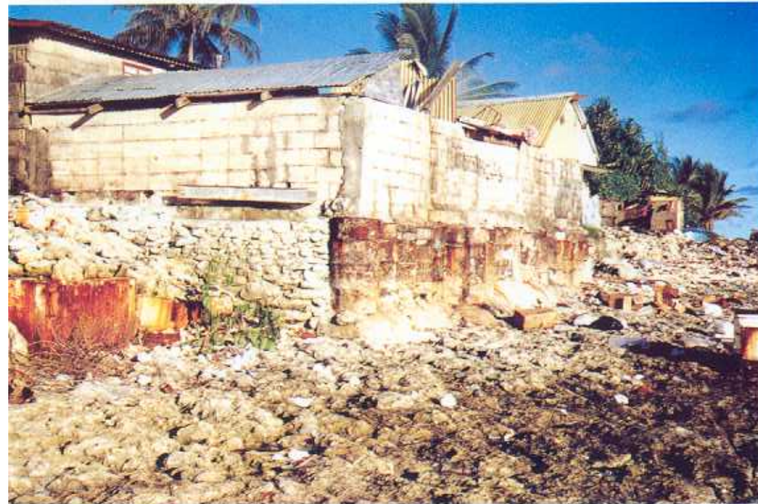
Plate 21. Vertical concrete block seawall and 44 gallon drums full of concrete protecting property on the ocean side reef flat of Majuro Atoll, Marshall Islands.
