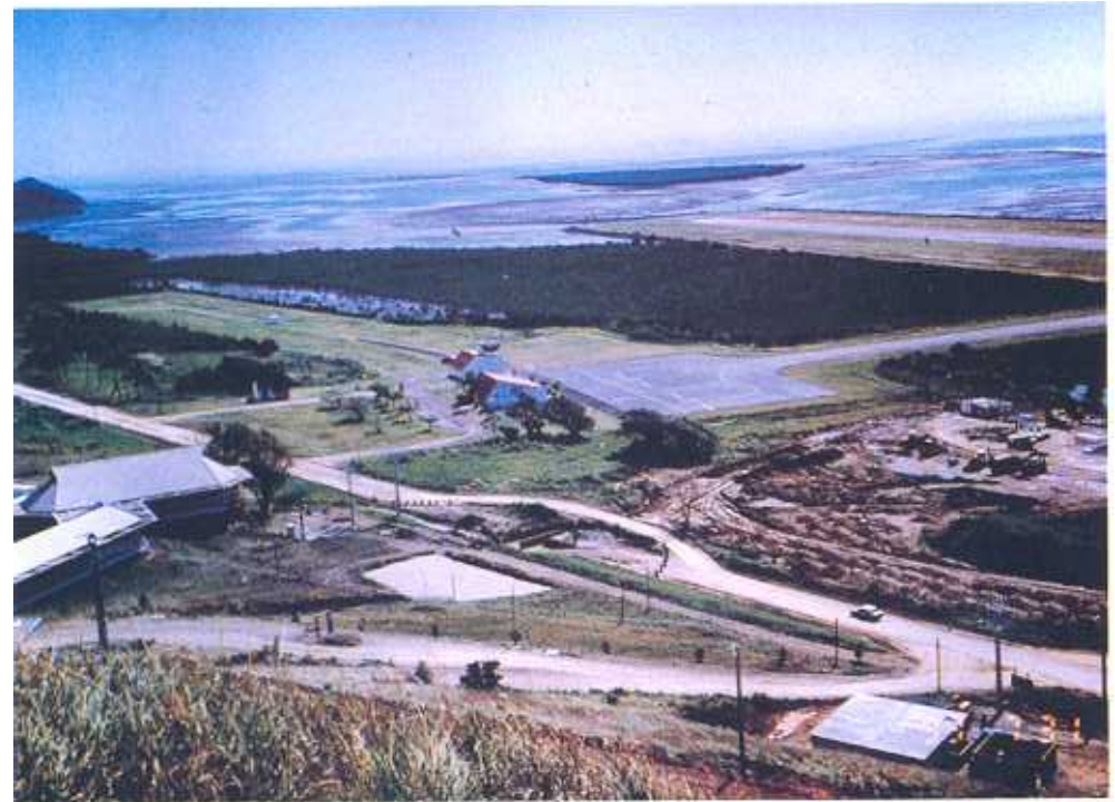
Plate 29. Touho runway, New Caledonia, reclaimed land on reef flat with mangroves along coast. Note position of old runway, also on reclaimed land.
