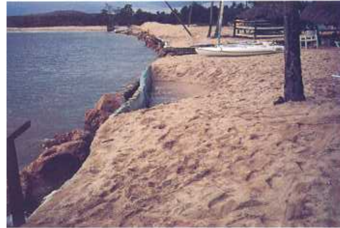
Plate 16. A beach forming part of a sand spit being eroded and threatening buildings at the Shangri-La Fijian Resort in Fiji. Note that attempts at protection using pine pole logs and large coral blocks do not appear to have been successful.
