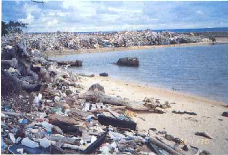
Plates 25 and 26. The present solid waste disposal site (rubbish dump) being retained by a wall constructed of gabion baskets on the ocean side reef flat of Majuro Atoll, Marshall Islands. Note the narrow reef flat and the position of the gabions virtually at the reef edge at the top right of Plate 25, above. The end result is useable reclaimed land (Plate 26).
