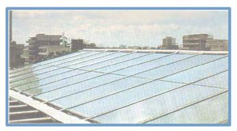
*Flat-Plate hydronic collectors* have a delivery temperature typically between 110 F and 160 F (43.3 C - 71.1 C). They are primarily appropriate for domestic water heating. They function using a thermosyphon, where natural circulation takes placed based on the density of hot or cold water. Efficiency is typically around 30% - 35%.
