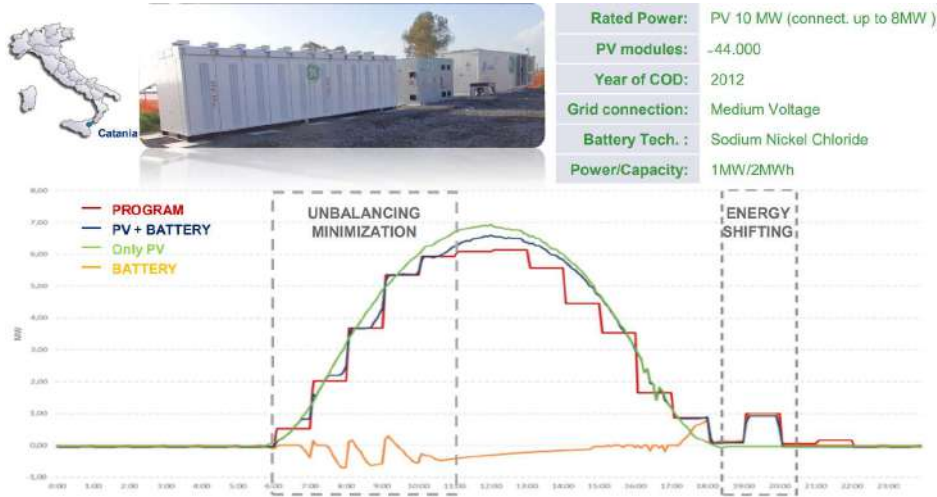
Figure 3.5: Solar Photovoltaic Installation with a Storage System
