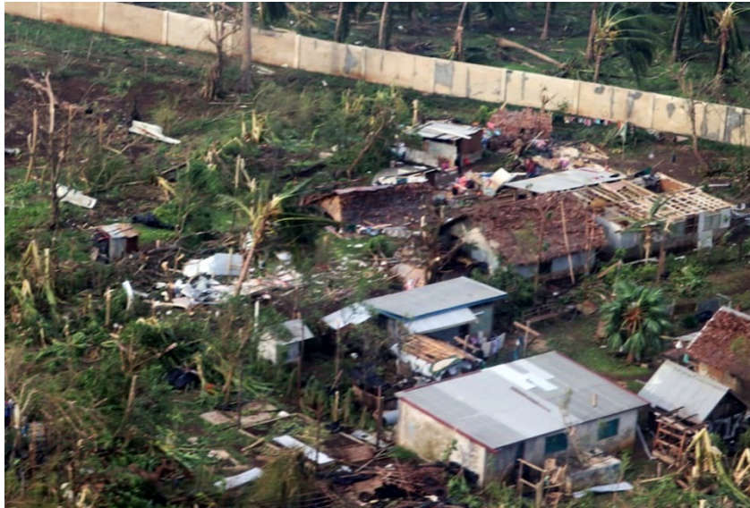
Figure 2: Many houses with thatch roofs survived in the cyclone (source: Tony Deamer).
