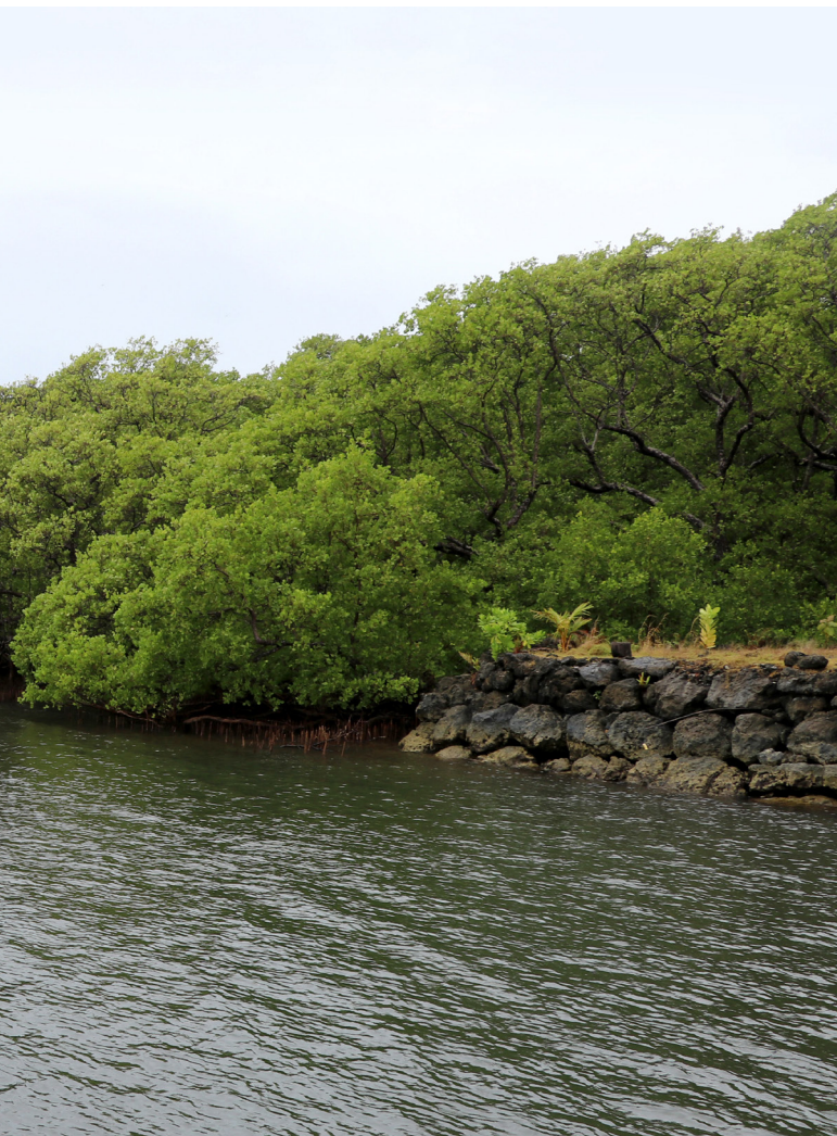
Traditional method: land reclamation integrating natural coastal protection, Yap, FSM. Photo: Greg Barbara
