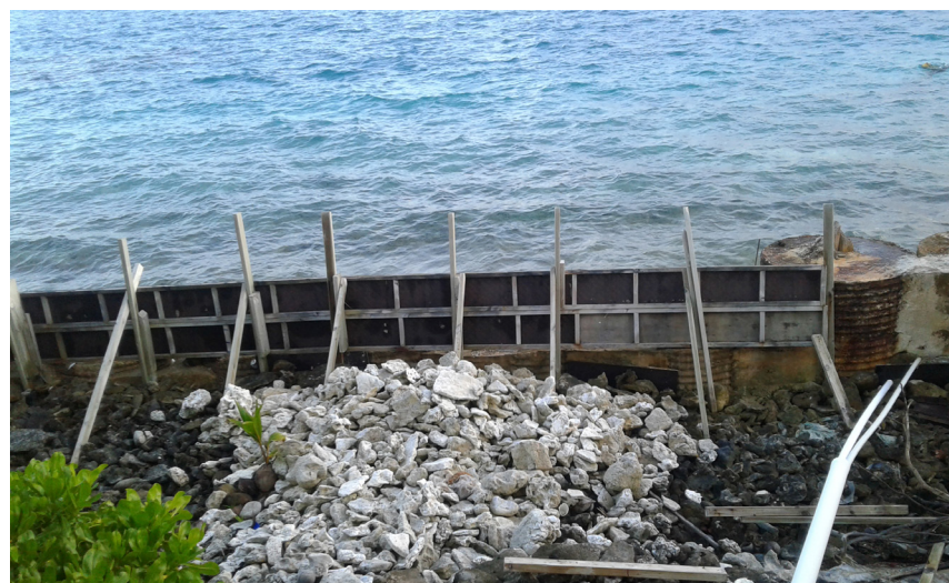
Adhoc coastal protection Nukunonu Atoll, Tokelau. Photo: Greg Barbara
