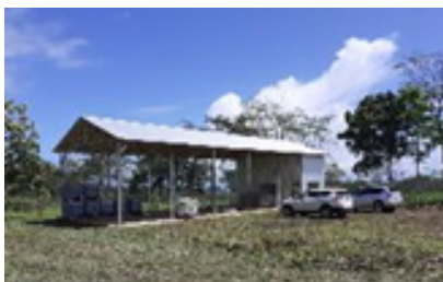
Construction of SWOMP facility completed, February 2021
