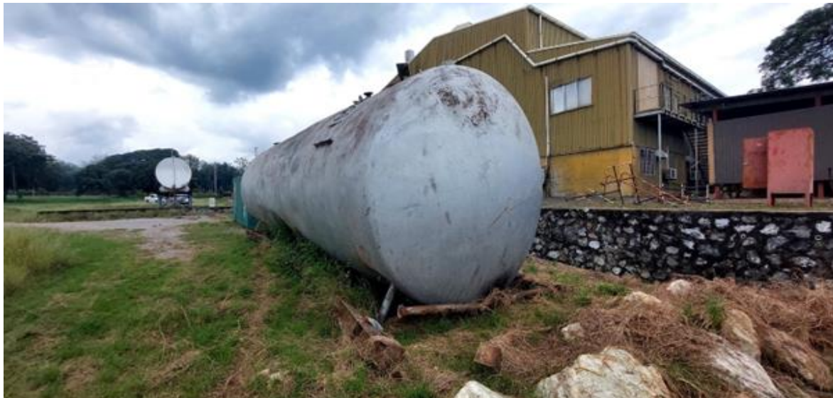
Figure 5: The remaining 20,000L of PCB contaminated oils are stored in this tank that is outside in the yard.
