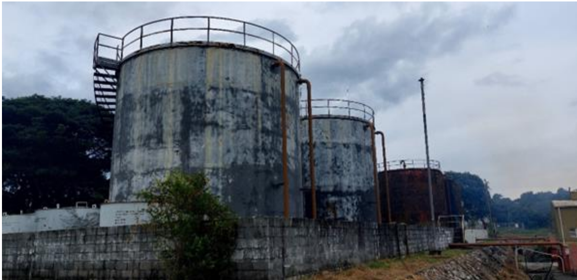
Figure 4: PCB contaminated oil is stored in Tank 1 estimated at 400 000L. The tanks are in a bunded area.
